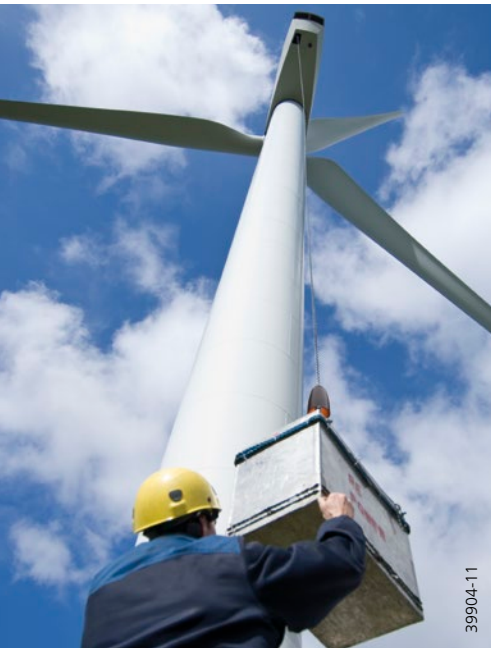
Up to 180 m hook path for the maintenance of wind turbines
