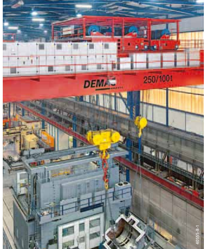
Process crane equipped with a 250-tonne MPW double hoist unit on a crab and a 100-tonne MPW open winch unit
